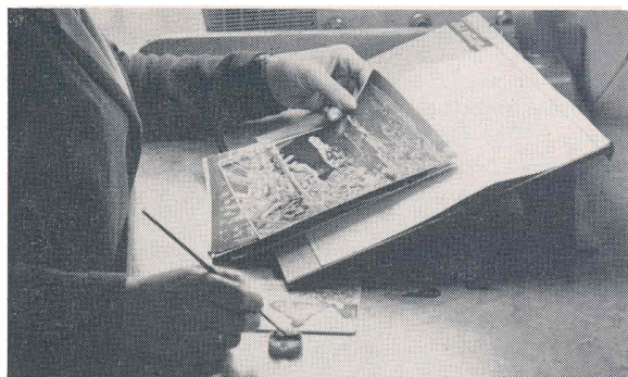
Touching brush to sponge (cut to fit small can lid) helps point brush and remove excess liquid. This is author's spotting set up at custom processing service.
