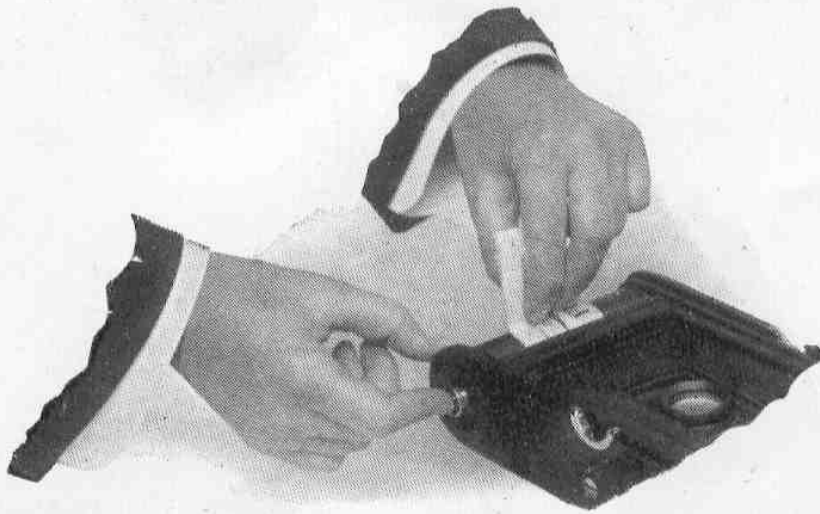
Fig. 4a. Pressing home the spool pins.
